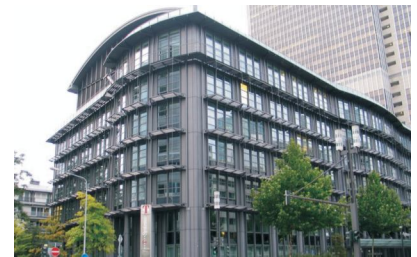
T Systems, Germany 41 TR (144 kW)
